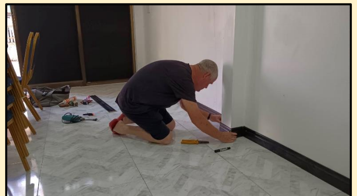
Ian installed baseboards in the worship room.
